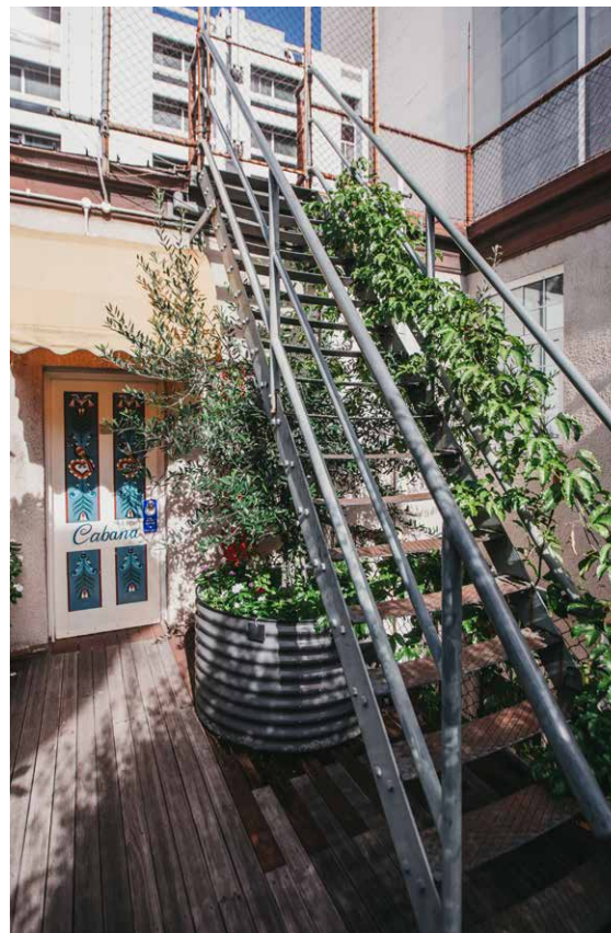
Planting on and underneath emergency stairs on rooftop
