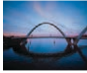
3 Queen Elizabeth Quay Bridge. Image courtesy of Sky Perth / City of Perth, 2018.
