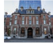
34-36 State Buildings. Image courtesy of City of Perth, 2017.
