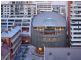
6 City of Perth Library
