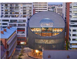
6 City of Perth Library
