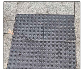
400X400X60 TACTILE PAVER - BLACKURBANSTONE WETCAST PAVER WITH PENETRABLE BREATHABLE SEALANT (DRYCRETE)
