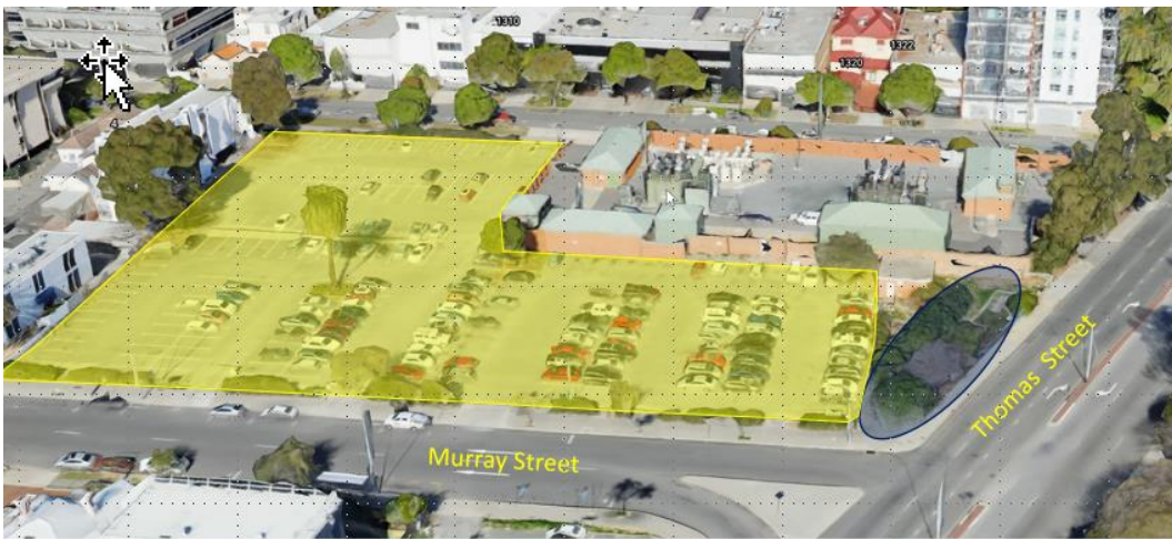
Existing pedestrian underpass location under Thomas Street
