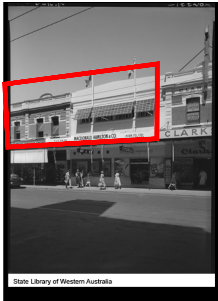
1956 Image showing extent of current screen and façades currently obscured (condition unknown)
