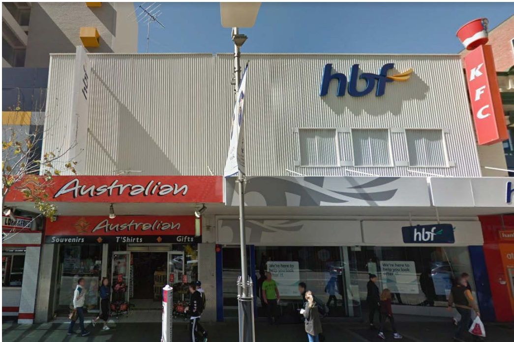
Current façade of 96 William Street
