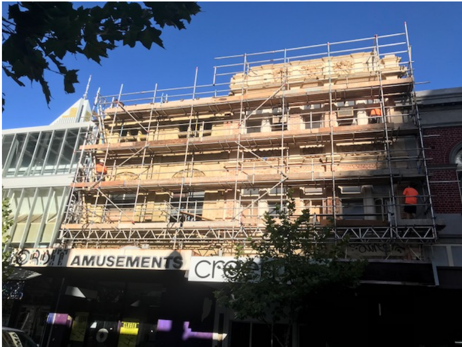
Screen removed and paint-stripping/restoration underway
