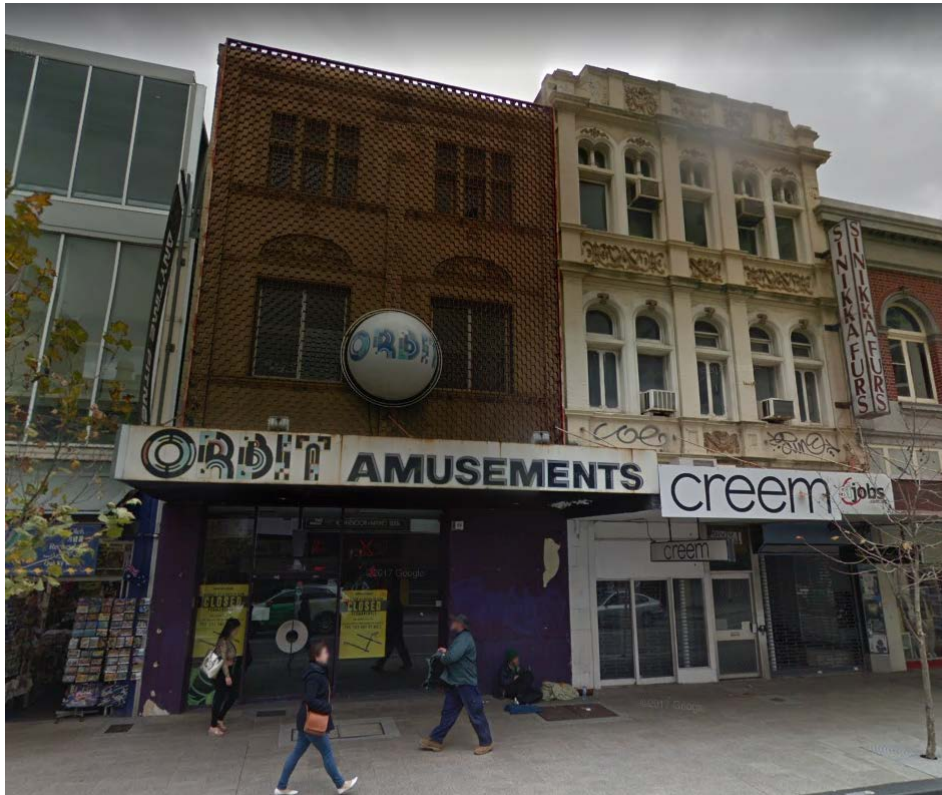
Prior to screen removal and restoration
