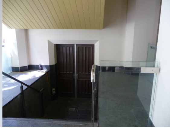
Figure 2: Existing Plant Room Stairwell
