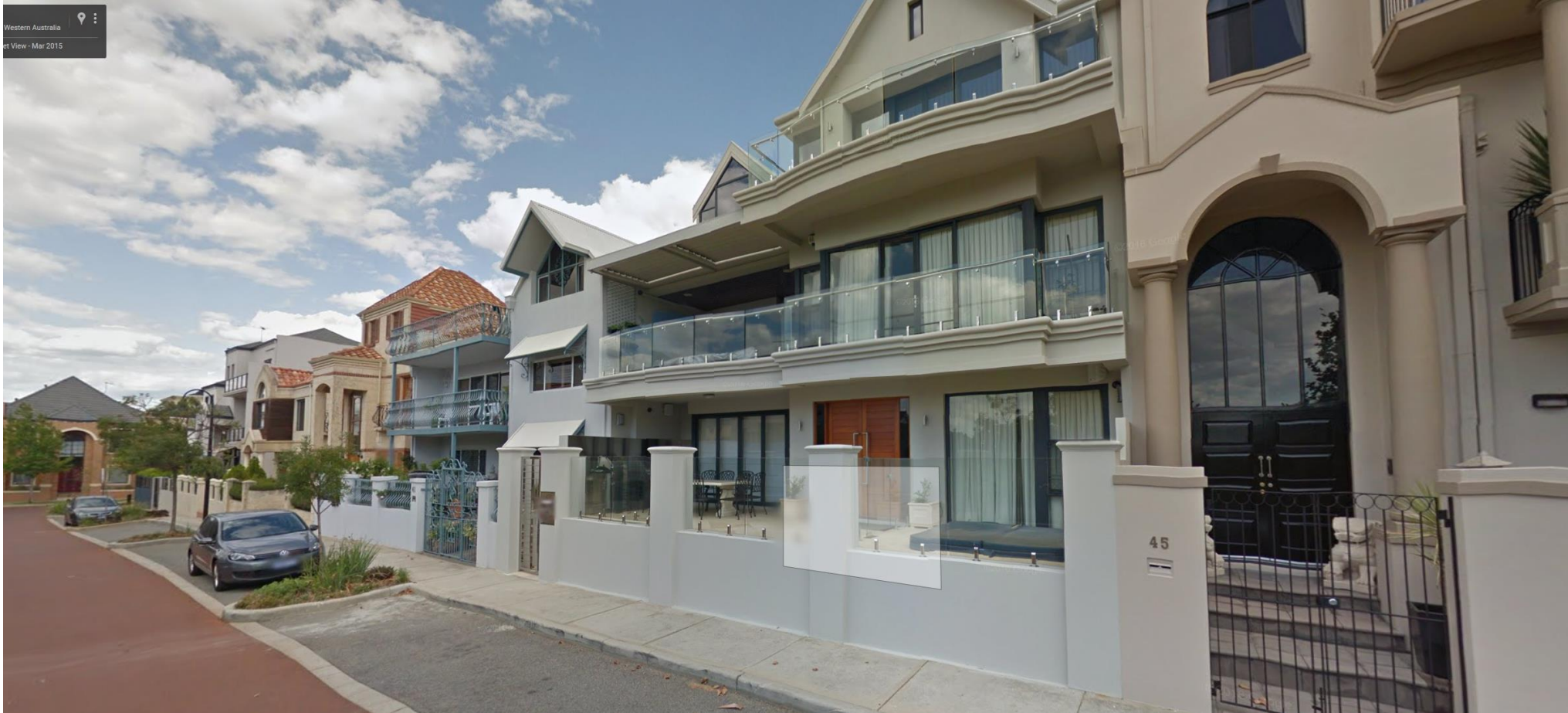
2016/5308 - 43 (LOT 41) ARDEN STREET, EAST PERTH (ARDEN STREET NORTH-WEST)
