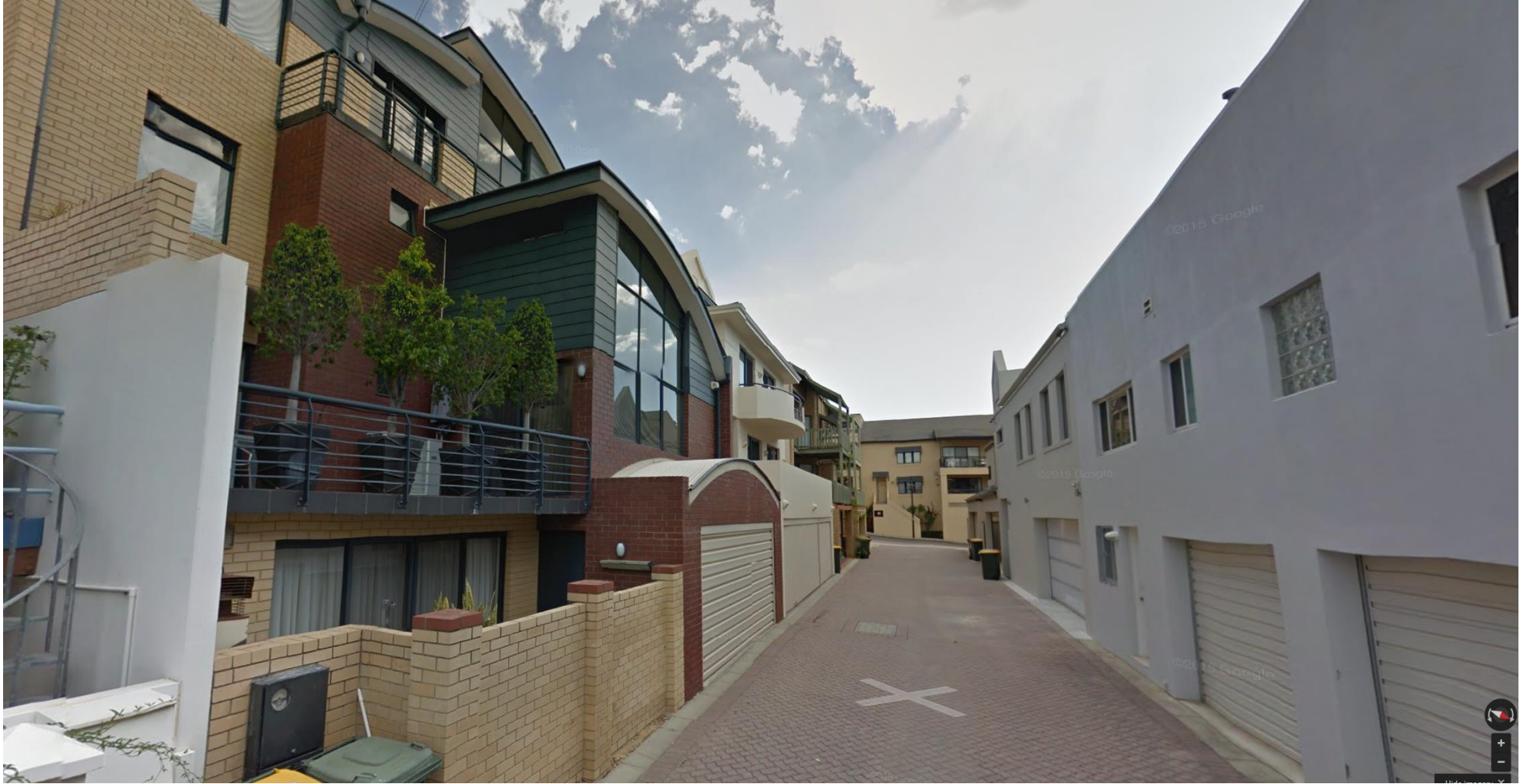
2016/5308 - 43 (LOT 41) ARDEN STREET, EAST PERTH (LANEWAY FROM EAST)
