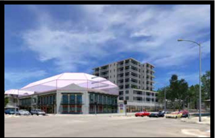
Plain Street looking south
