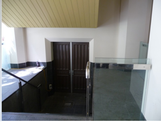
Figure 2: Existing Plant Room Stairwell
