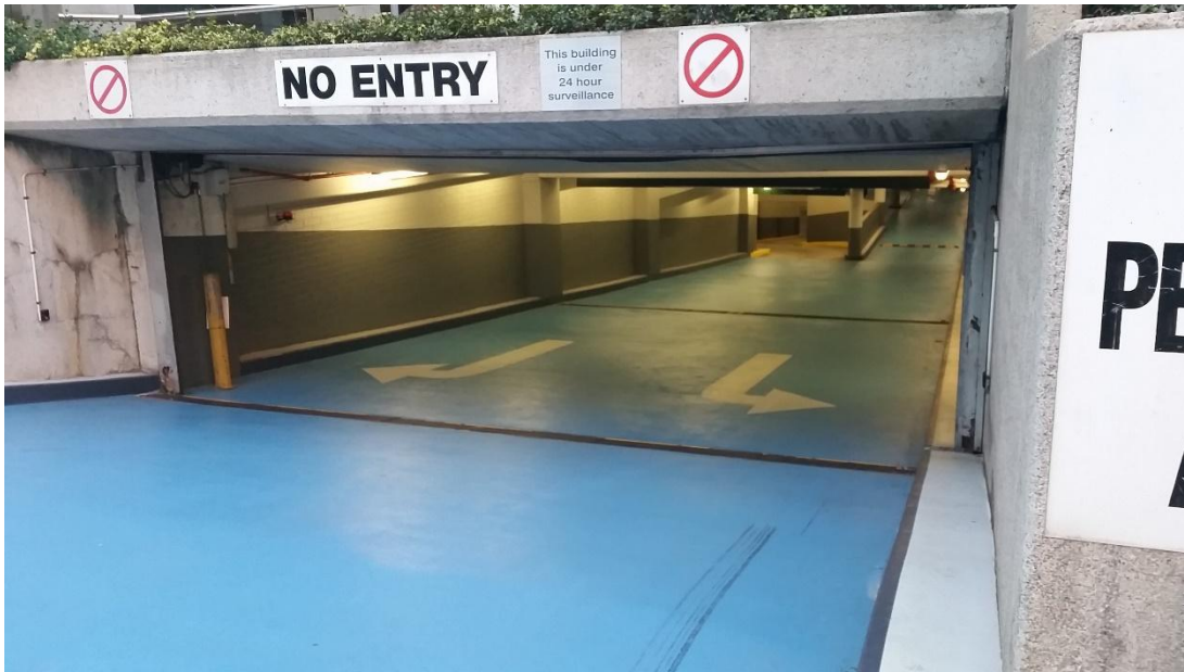
Figure 2.3 Central Park Carpark exit at 17:00
