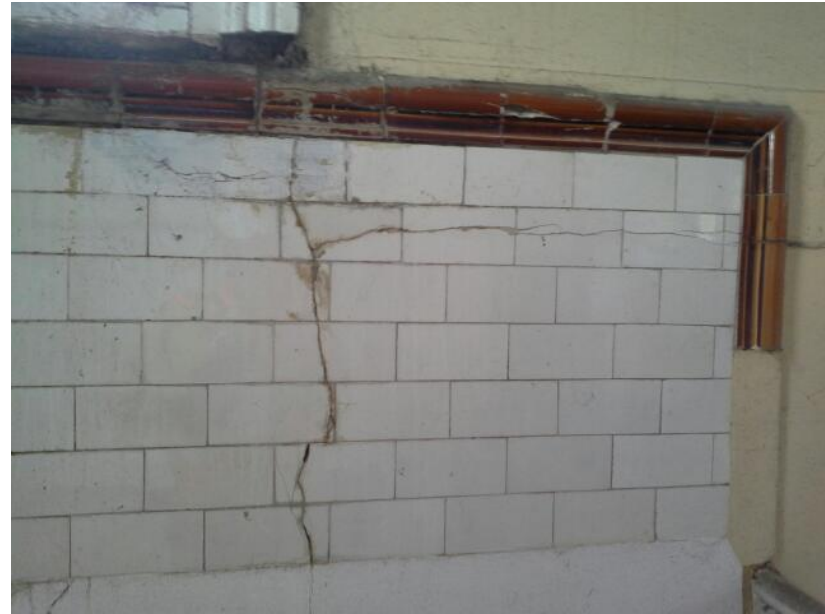
Photograph 12 Typical Cracks to interior walls
