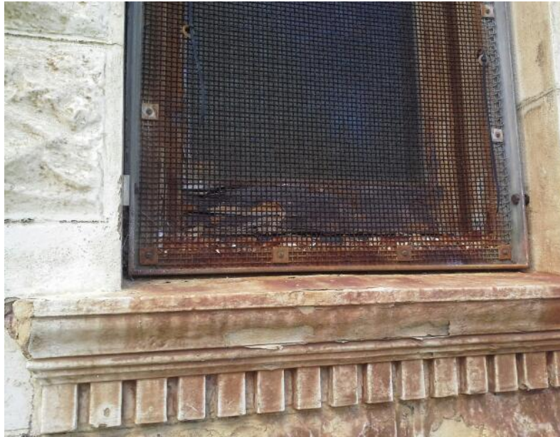
Photograph 11 Deterioration of exterior Window Frame Western End
