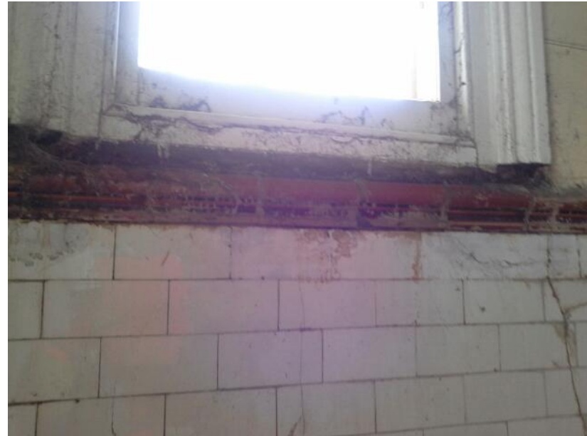
Photograph 10 Deterioration of Window Frame
