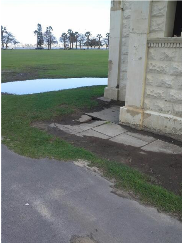
Photograph 9 Damage to Pavement on South Eastern corner of building
