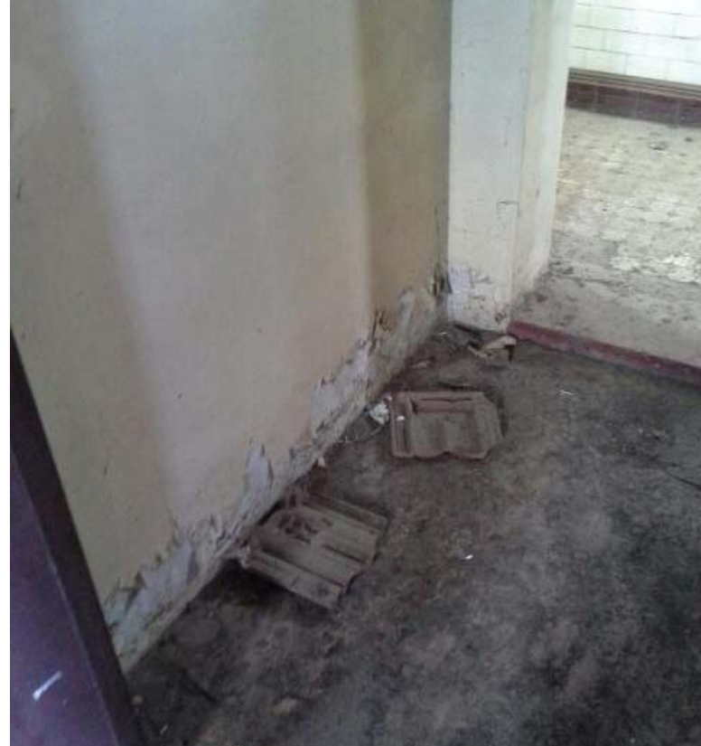
Photograph 8 Water Damage around base of wall
