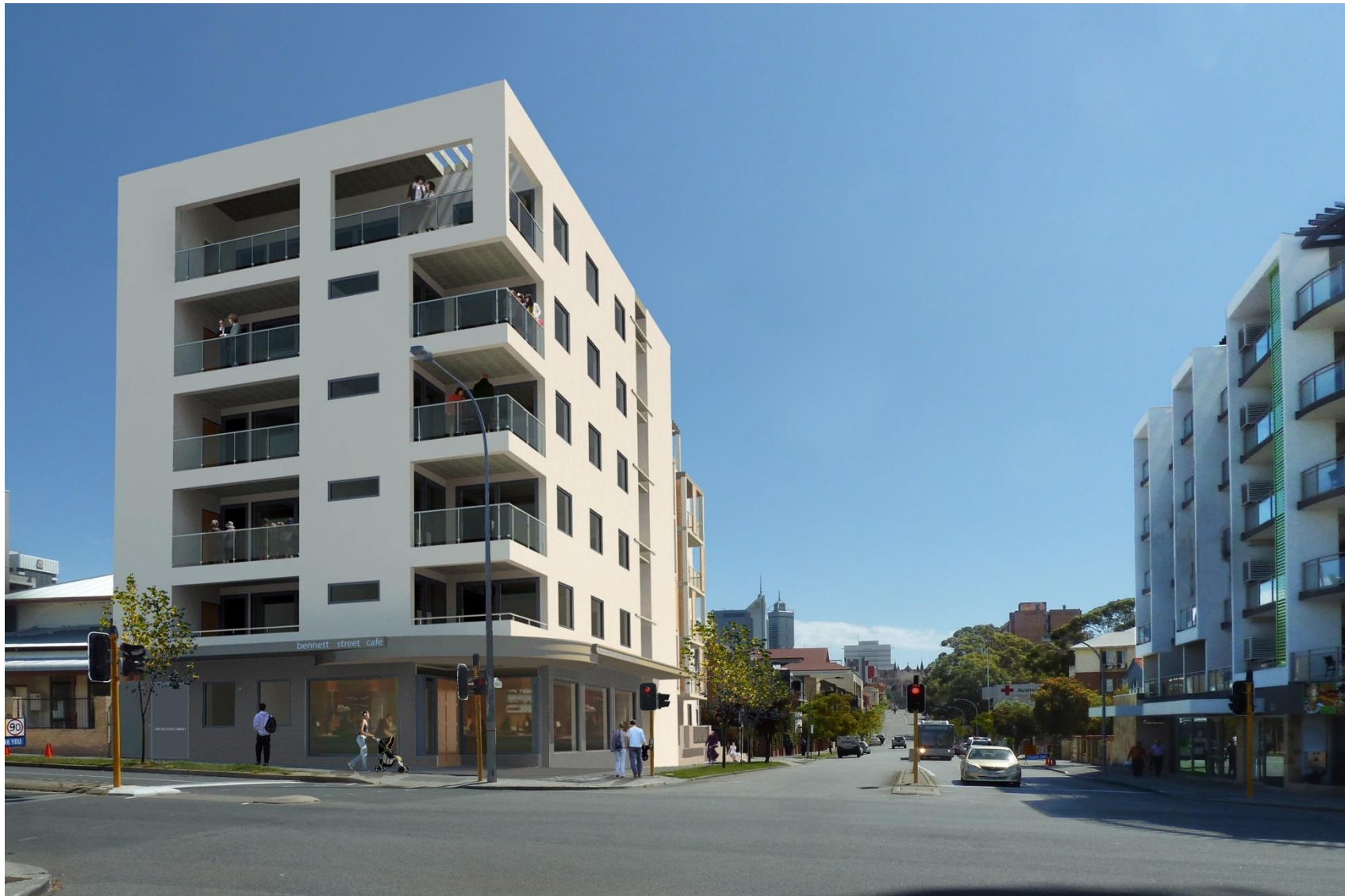
2014/5287: 61-61A BENNETT STREET, EAST PERTH
