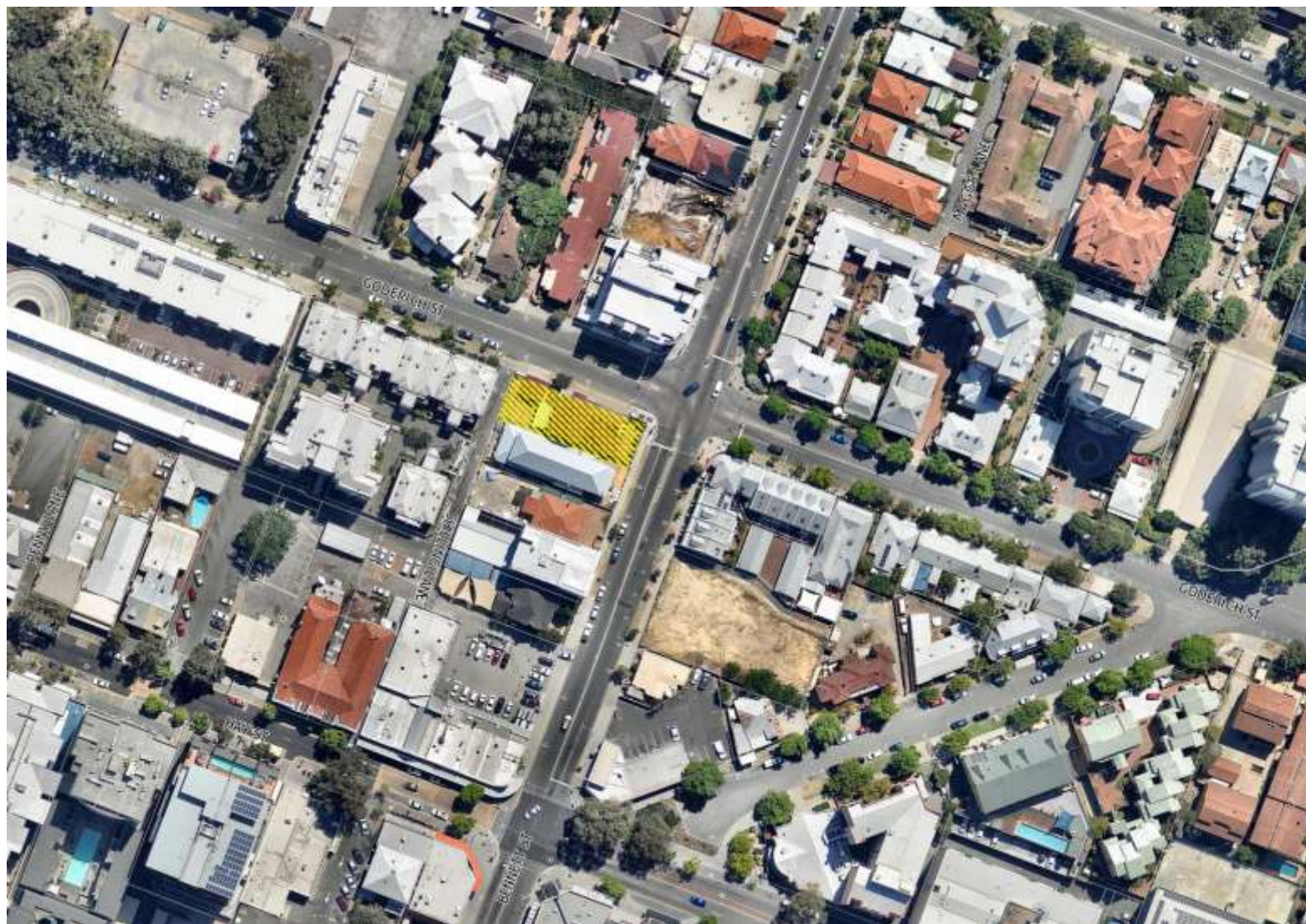
2014/5287: 61-61A BENNETT STREET, EAST PERTH
