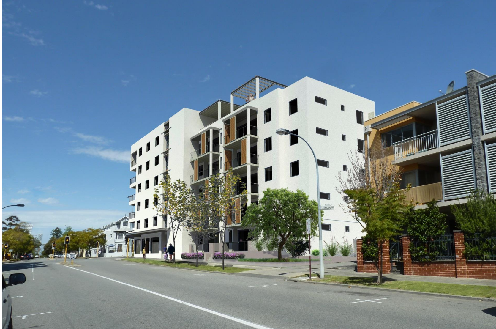
2014/5287: 61-61A BENNETT STREET, EAST PERTH
