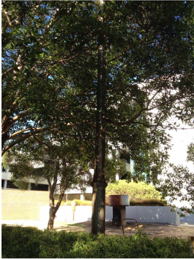
P23762 Sewerage Vent, East Perth ; View from Royal Street looking southwest ; Sian Ferraz 06 Feb 2012
