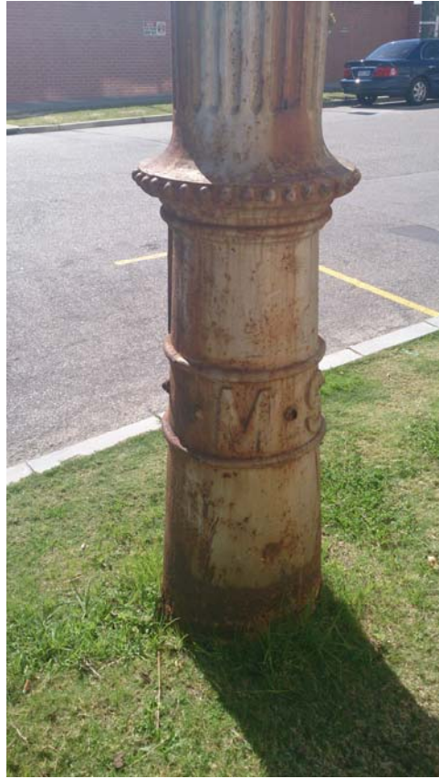
P23782 Sewerage Vent, Princess Margaret Hospital, West Perth ; View of Cast Iron base showing 'M.S' lettering ; Sian Ferraz 21 Aug 2013
