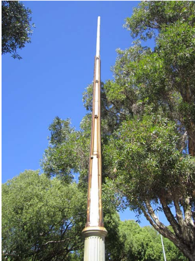
P23738 Sewerage Vent, West Perth ; Detail; support structure and top of vent ; Karina Williams 07 Feb 2014
