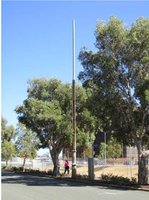
P23738 Sewerage Vent, West Perth ; View across Arthur Street, looking north ; Karina Williams 07 Feb 2014
