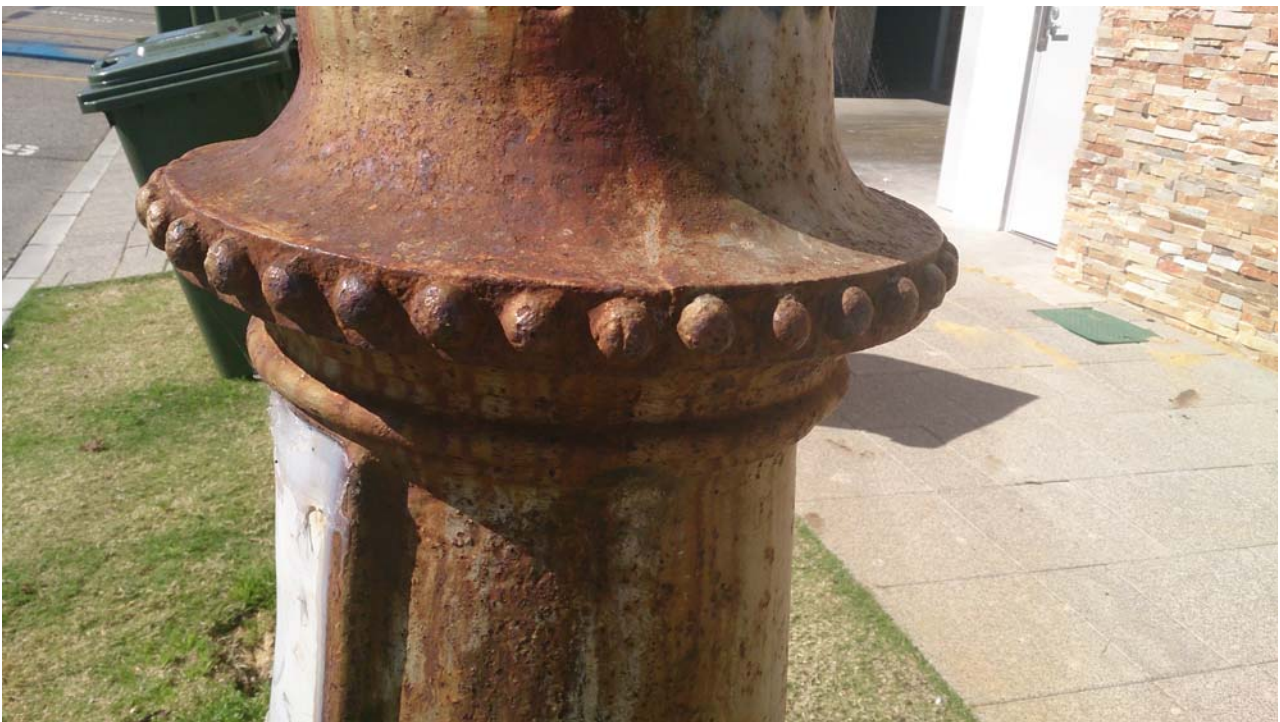
P23782 Sewerage Vent, Princess Margaret Hospital, West Perth ; Detail of Cast Iron base ; Sian Ferraz 21 Aug 2013
