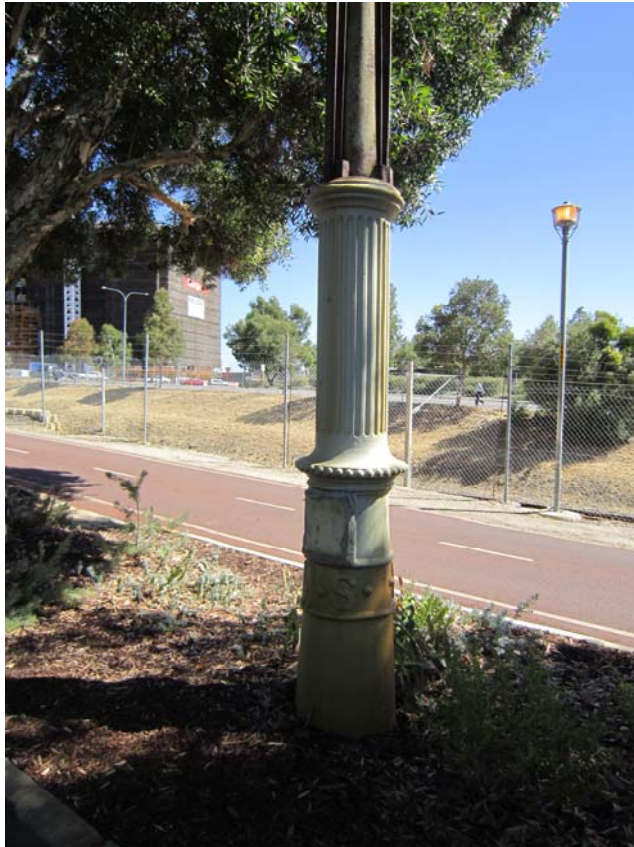
P23738 Sewerage Vent, West Perth ; Detail; Cast iron base ; Karina Williams 07 Feb 2014
