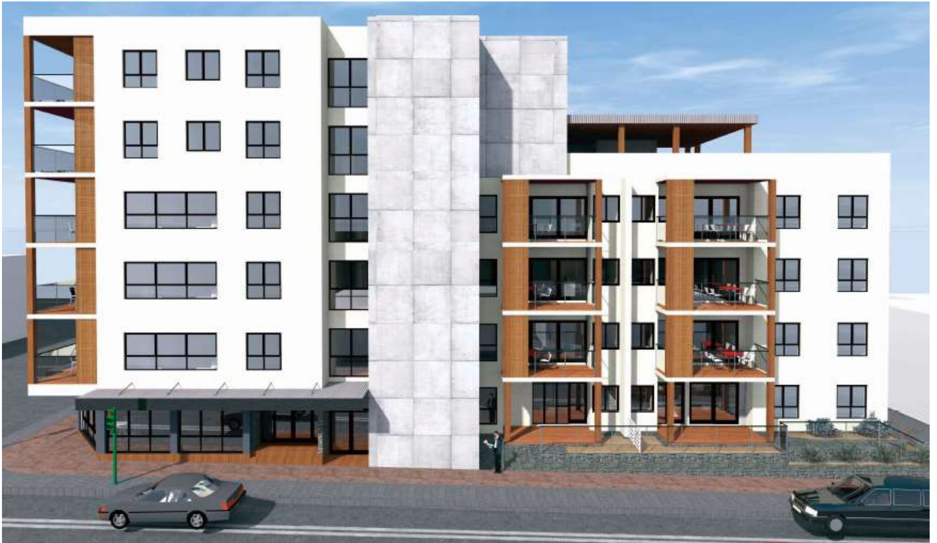
2014/5287: 61 -61A BENNETT STREET, EAST PERTH
