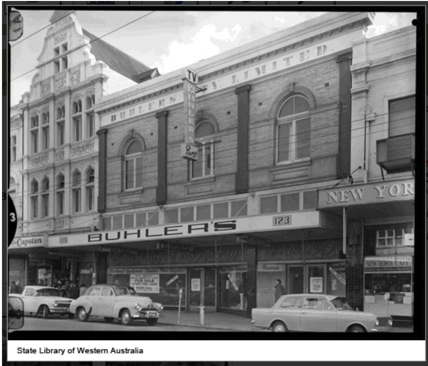
ORIGINAL TO BE REINSTATED
