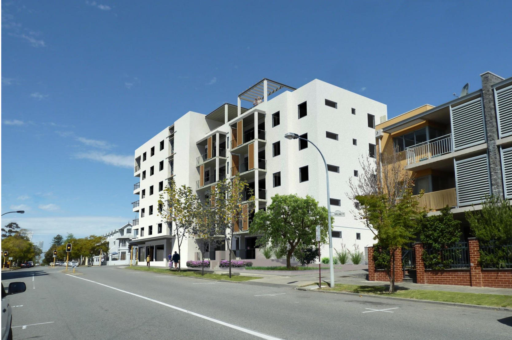
2014/5287: 61-61A BENNETT STREET, EAST PERTH
