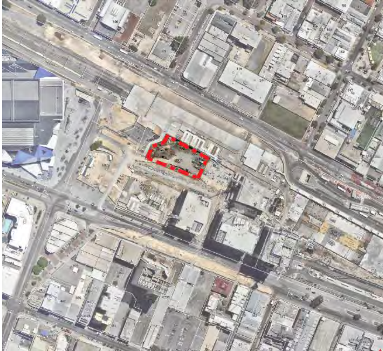
2015/5118; KS6, 566 (LOT 9000) WELLINGTON STREET, PERTH
