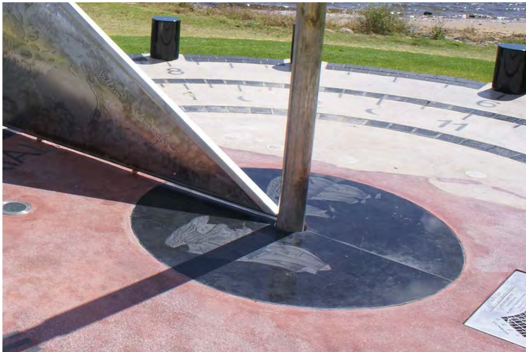
Clock Face Centre-piece - laser etched ship images on polished granite 2
