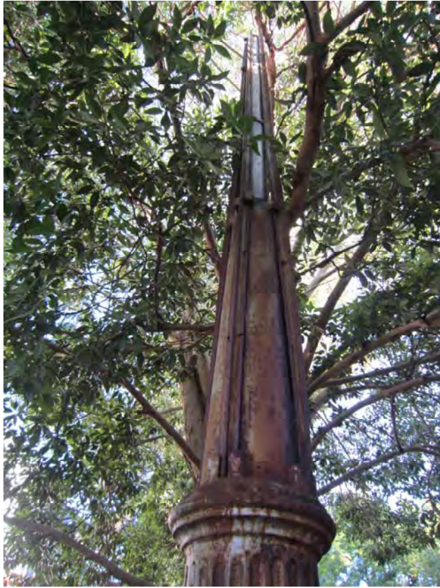
P23762 Sewerage Vent, East Perth ; Steel support brace to ventilation pipe ; Karina Williams 06 Feb 2014
