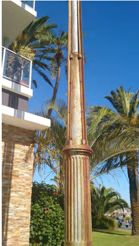
P23782 Sewerage Vent, Princess Margaret Hospital, West Perth ; View of Cast Iron base and vent pipe ; Sian Ferraz 21 Aug 2013
