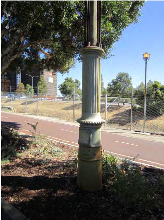
P23738 Sewerage Vent, West Perth ; Detail; Cast iron base ; Karina Williams 07 Feb 2014
