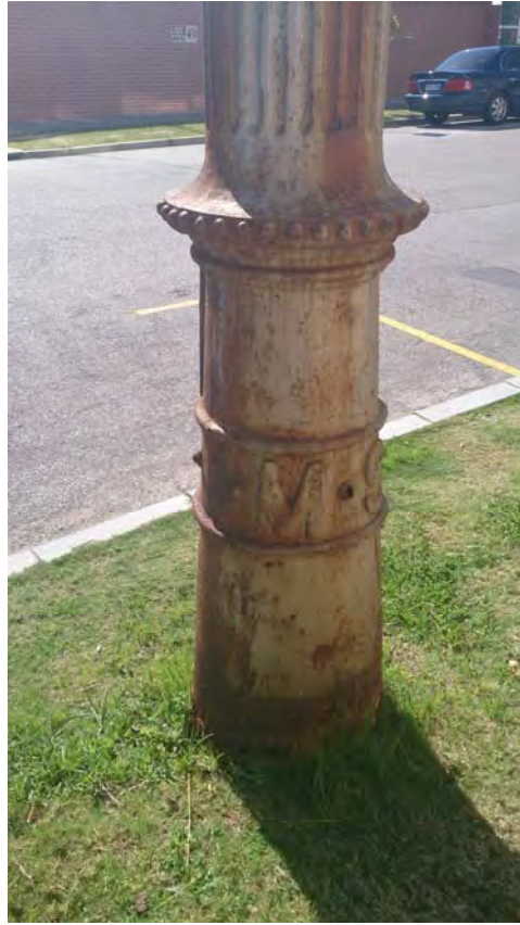
P23782 Sewerage Vent, Princess Margaret Hospital, West Perth ; View of Cast Iron base showing 'M.S' lettering ; Sian Ferraz 21 Aug 2013
