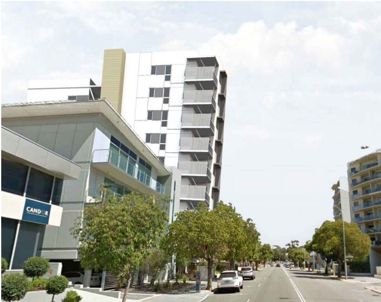
2014/5344: 989 WELLINGTON STREET, WEST PERTH
