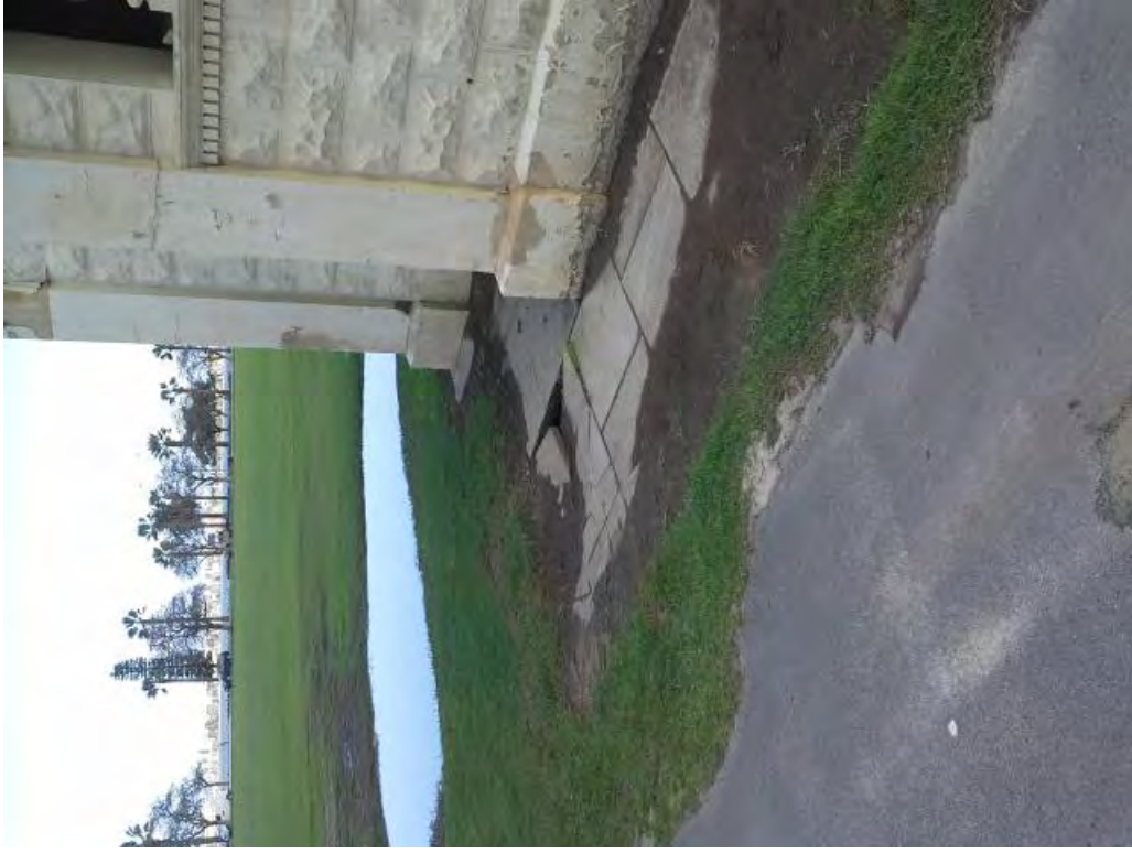
Photograph 9 Damage to Pavement on South Eastern corner of building
