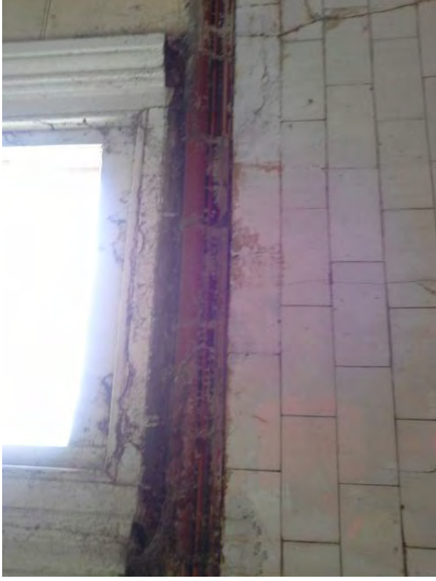
Photograph 10 Deterioration of Window Frame
