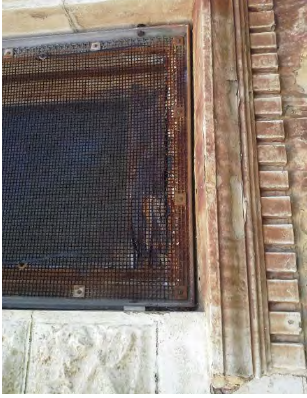
Photograph 11 Deterioration of exterior Window Frame Western End
