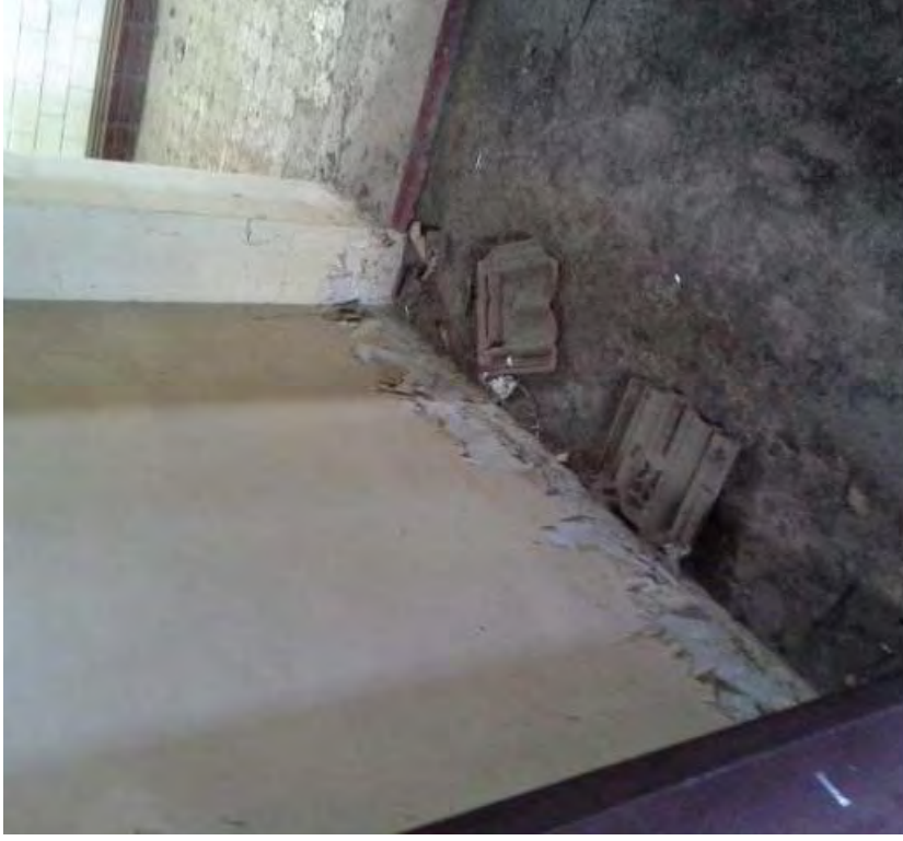
Photograph 8 Water Damage around base of wall
